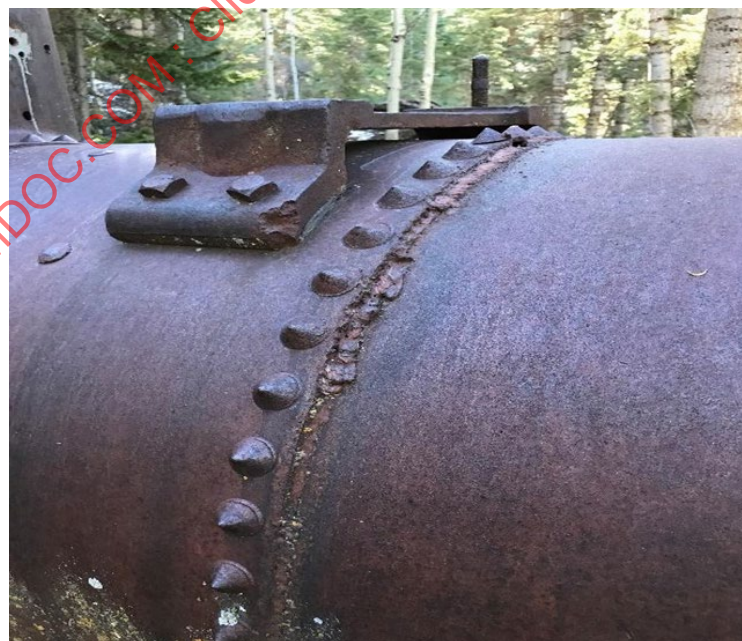
Figure 1-1: Period Repair Work on a Riveted Seam
