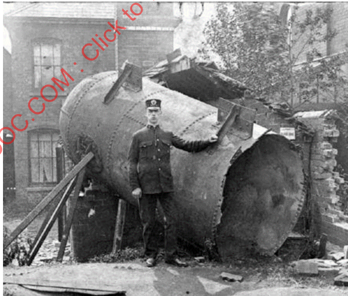
Figure 1-3: Policeman Next to Another Failed Boiler
