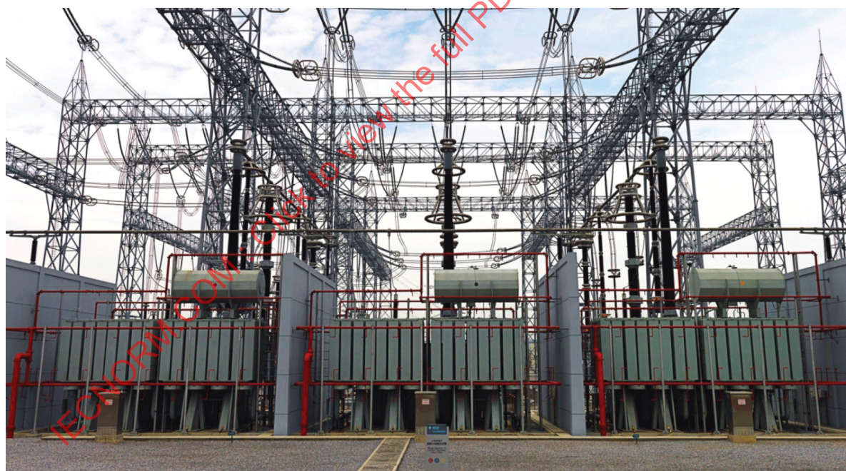
Figure C.2 – UHV AC shunt reactor
