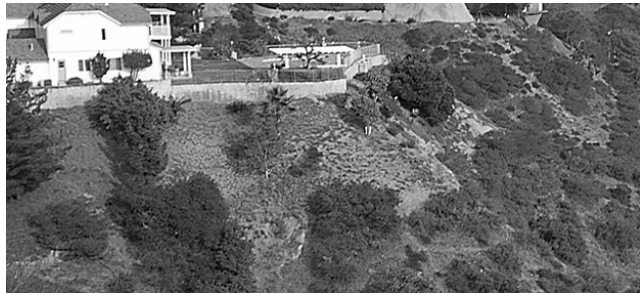
FIGURE A.5.1.3.3(a) Noncombustible Barrier on the Edge of a Downslope. (Courtesy of Firewise Communities Program. Photo by J. Smalley.)
