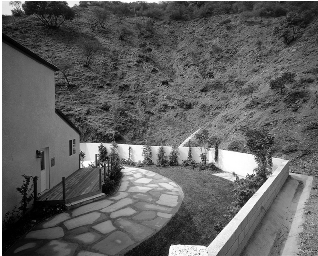
FIGURE A.5.1.3.3(b) Noncombustible Barrier Behind a House on the Edge of the Upslope. (Courtesy of Firewise Communities Program. Photo by J. Smalley.)
