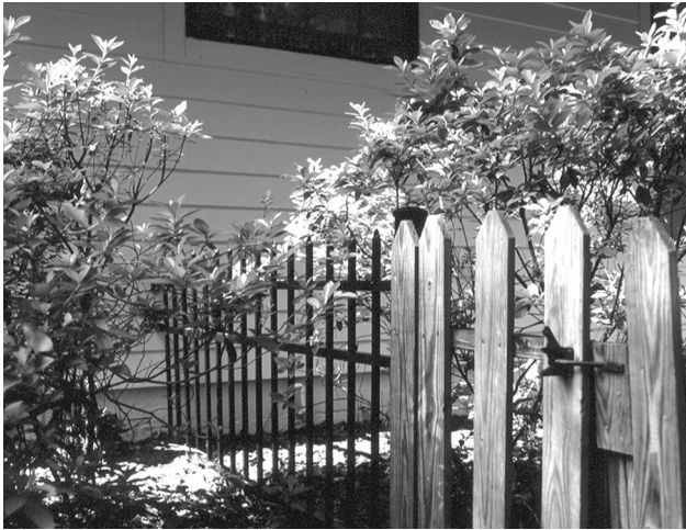
FIGURE A.4.2.4.3(b) Transition Fence Separates Combustible Fence from Structure. (Courtesy of Firewise Communities Program. Photo by G. Johnston.)
