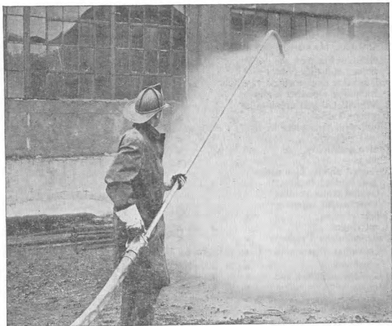
A-11.31. Spray nozzle in operation on a typical applicator.
