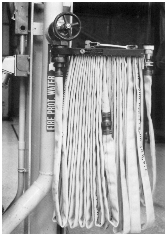
FIGURE A.4.2 Typical Standpipe and Fire Hose Rack Arrangement. (Courtesy of National Aeronautics and Space Administration.)
