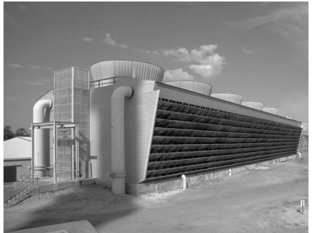
FIGURE B.1(e) Typical Induced-Draft Crossflow Water-Cooling Tower.
