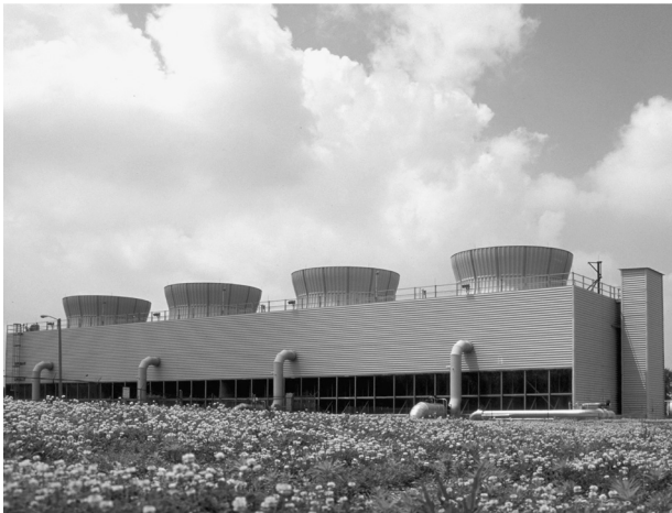
FIGURE B.1(d) Typical Induced-Draft Counterflow Water-Cooling Tower.
