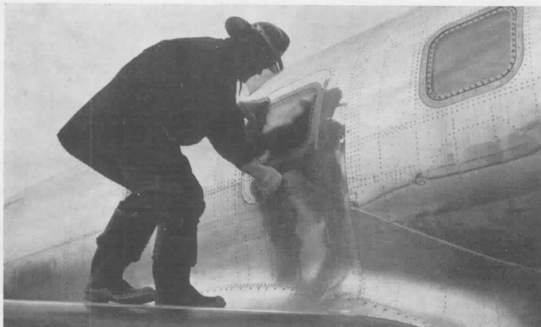
Figure A-18. The fourth window from the front on each side of the JetStar fuselage is an emergency hatch. To open from the outside, push in on the bottom of the flush latch plate underneath the bottom edge of the window. Push inward.
