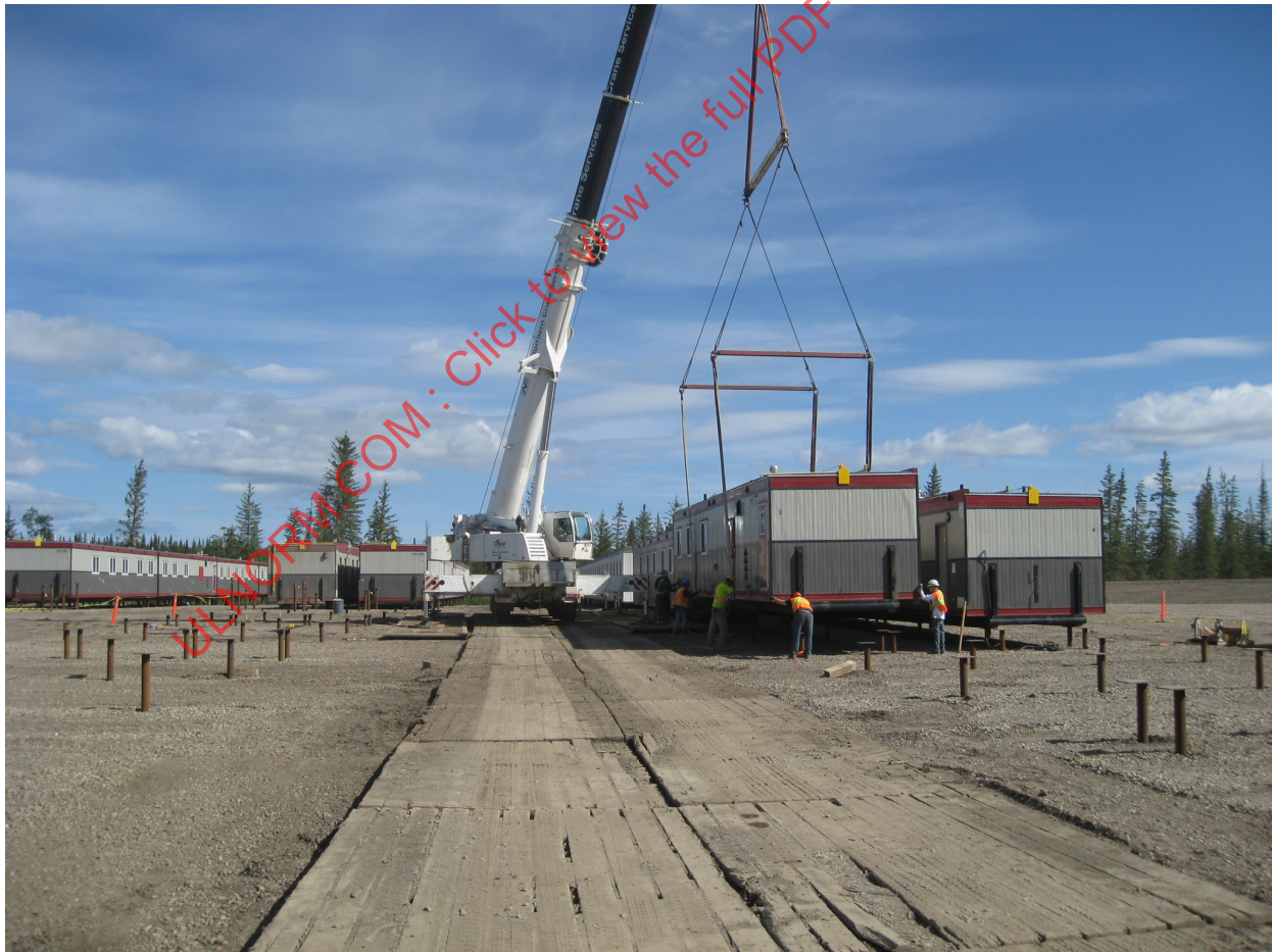
Figure C7.2 Dormitory Units on Screw Piles
