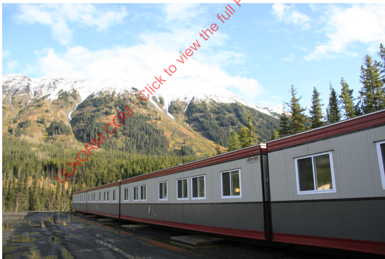
Figure C7.2.1 Dormitory building on rig mats
